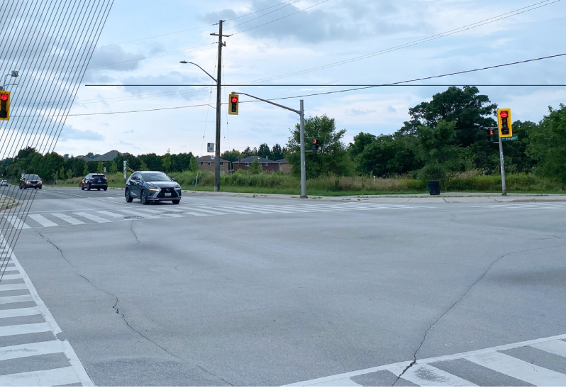
Photo 1: South of the subject corridor, this street has an urban cross-section with three lanes of traffic (one through-lane in each direction plus a centre turning lane), on-road bike lanes, and sidewalks on both sides of the road.
