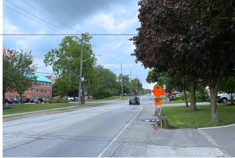
Photo 2: Within the southern portion of the subject corridor, this street has a two-lane rural cross-section with a sidewalk on the west side.
