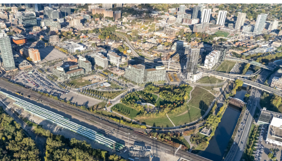
Aerial view of Corktown Common, the new park that was built as the first phase of flood protection for the eastern waterfront. It unlocked the area now known as the Canary District for development of a new neighbourhood.
