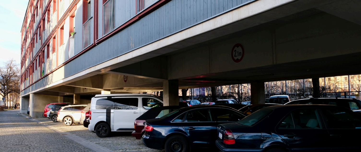
Figure 2: The Dantebad social housing project in Munich has created 100 housing units. By building the housing on pillars above the parking lot, 105 of the 111 parking spaces have also been retained. Photo by George Liu
