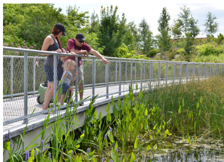
The wetland in Corktown Common is part of its design for stormwater management. It also provides diverse natural habitat.
