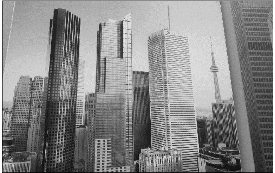
The Trump International Hotel and Residences, shown in the centre, has a much higher density, but similar built form and scale to its neighbours, Scotia Plaza and First Canadian Place
