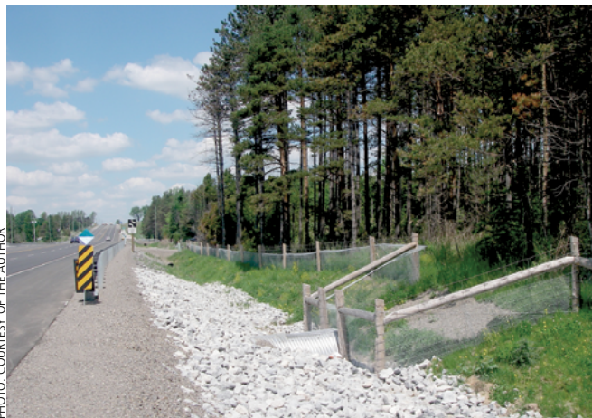
Exclusion fencing and ecopassage installed by MTO on Highway 10 to protect turtles
