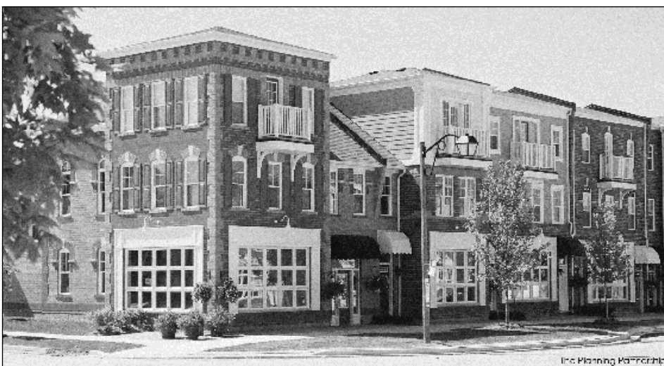
Units are pre-zoned to allow commercial use
