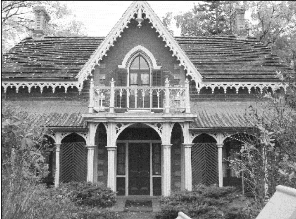
Hillary House, National Historic Site, now a museum, which is located in the Heritage District
