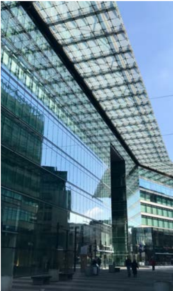
Continuous weather protective awning in Berlin
