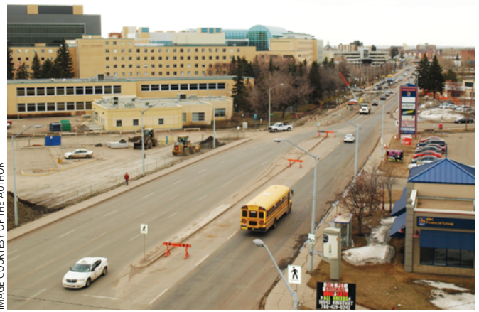
Relocation of utilities in anticipation of 2011 construction season on the North LRT, Edmonton
