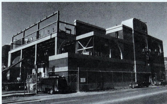
Esplanade Transformer Station
