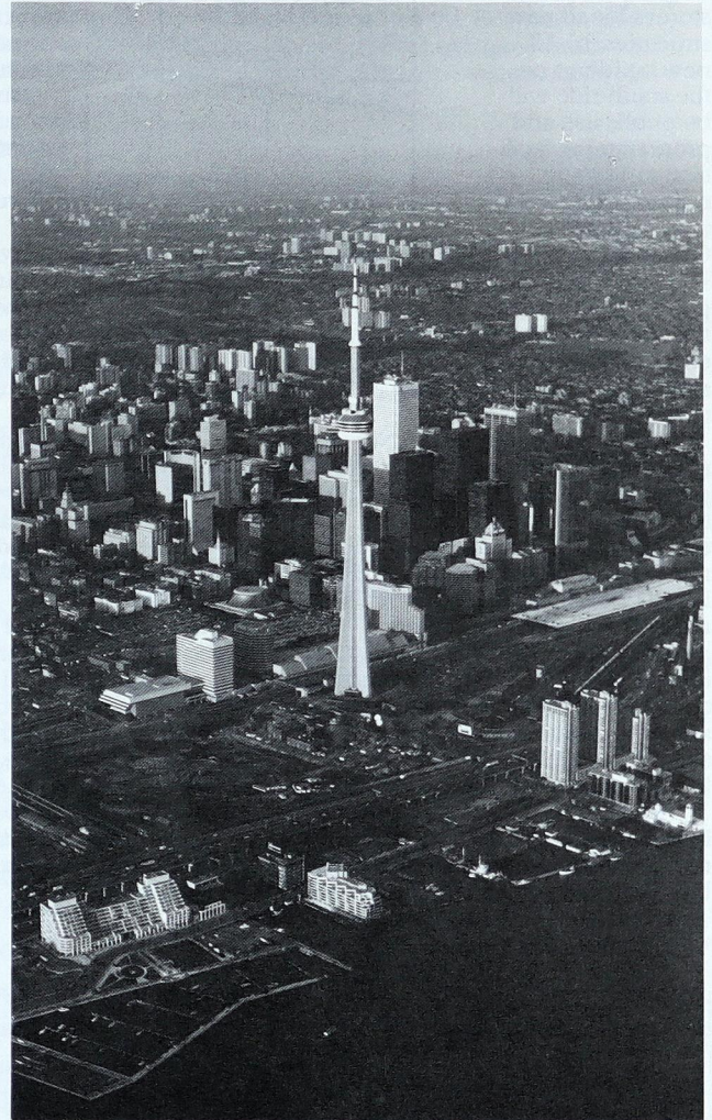
King's Landing (left) and Harbourpoint (3 towers), dominate Harbourfront
