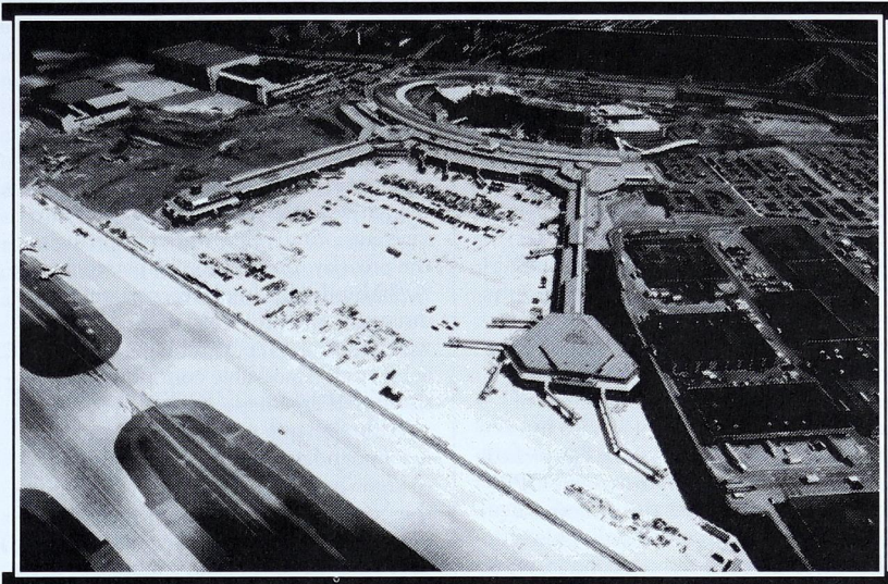
The nearly completed Terminal Three Building: future privatization initiatives at Pearson may hinge on the government's experience with this project.
