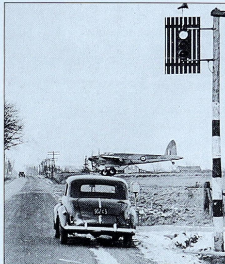
Airfield / signalized intersection at Dufferin St. before it was closed in the 1940s
