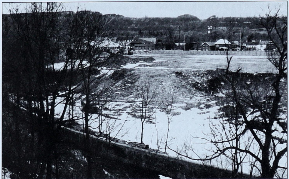
Filling in the holes in the urban fabric
