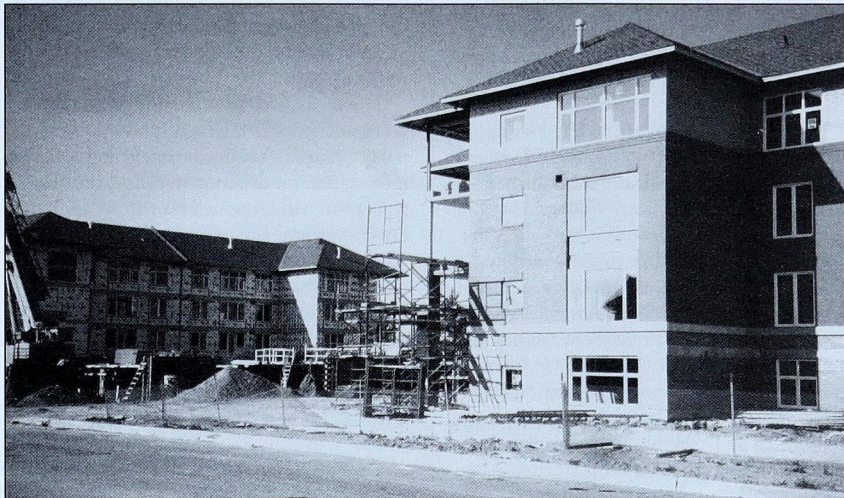
The Meridian under construction in Nepean
