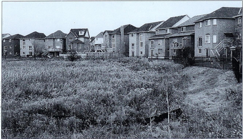
New residential lots backing onto wetland EPA formerly known to support migratory amphibian populations. Note limit of grading immediately at edge of wetland
