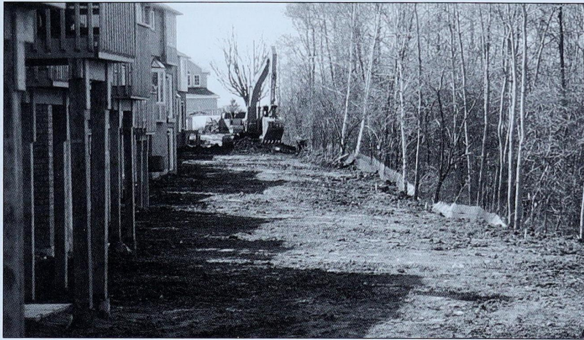
Townhouse development backing onto wooded EPA with no buffer. Footprint of residential use will extend well into the EPA. Note depth of fill against/over top of sediment control fence. OPA 129 lands in Richmond Hill
