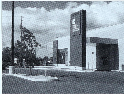
This Bank of Montreal at the intersection of Trafalgar & Dundas in Oakville in a retail plaza is located to address the urban corner appropriately. The drive-through stacking lane is contained within the site without any negative impacts
